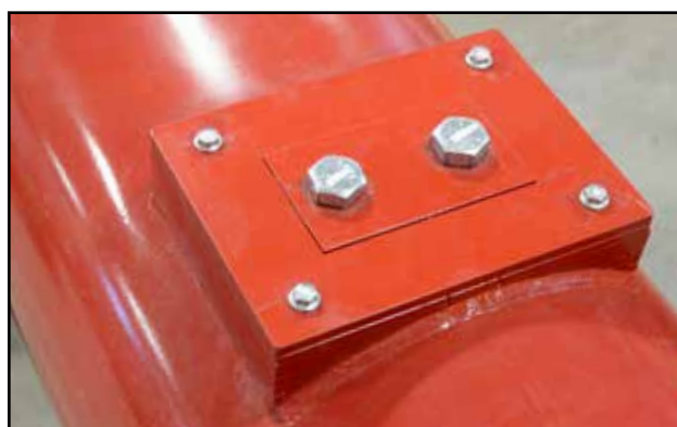
Fig 47 - Cover Plate covering Hanger Bearing
